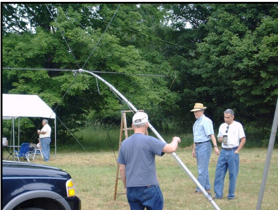
Field Day 2003 Antenna Crew Raising the 20 Meter Hex Beam
